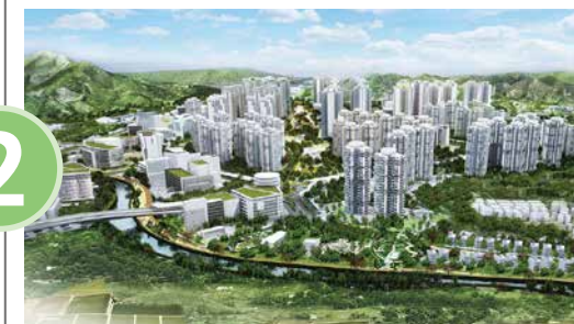
Public Housing Development at Kwu Tung North Area 19 Phase 2 – Sun Fook Kong 古洞北第19區第二期公營房屋發展 – 新福港
